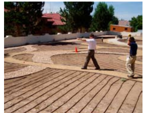
Site inspection of walk layout, and planting beds
