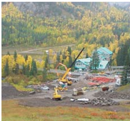
Lodge and Spa under construction
