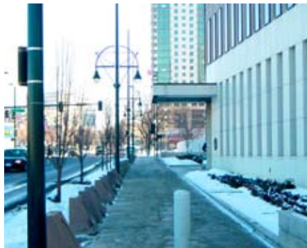
20th Street after renovation
