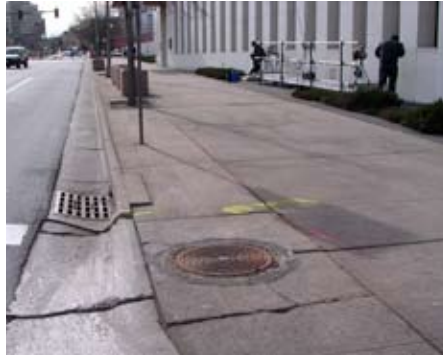
20th Street before renovation
