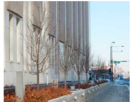
Champa Street after renovation
