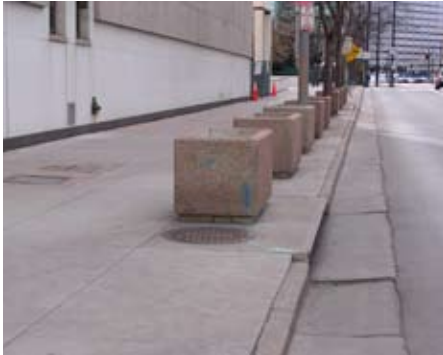
19th Street before renovation
