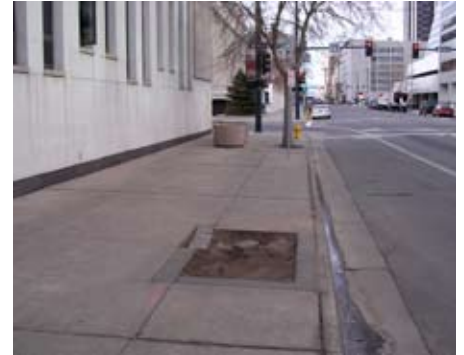
Champa Street before renovation
